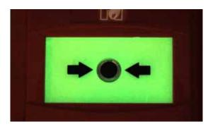
A special photo luminescent pigment is incorporated within the white plastic operating window. In the event of a power failure or reduced light conditions the call point will remain visible for approximately 5 minutes to assist building occupants in locating the unit.
