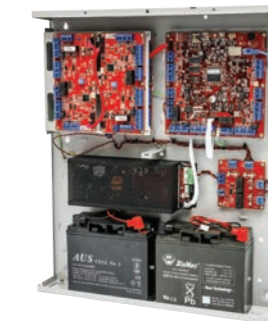
IAC Controller shown in 8 Door configuration. Housed in a WideBody Enclosure with 8Amp SMART Power Supply & 3 x UniBus Door Expanders. (IK-996035WB8PS Kit)
