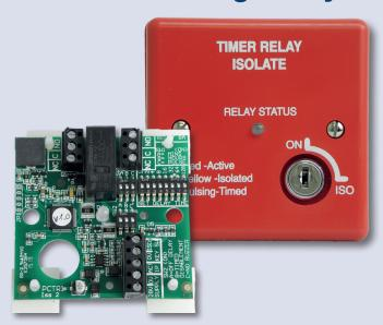
The timer relay unit is configurable to provide a variety of operational functions which are determined via DIL switch settings.
