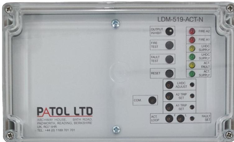
The ACT-N controller is designed to monitor a zonal length of Analogue Linear Heat Detection Cable (LHDC) for elevated temperature states. Two adjustable levels of alarm are provided (A1 & A2), one of which may be optionally employed as a “Pre-Alarm”.
